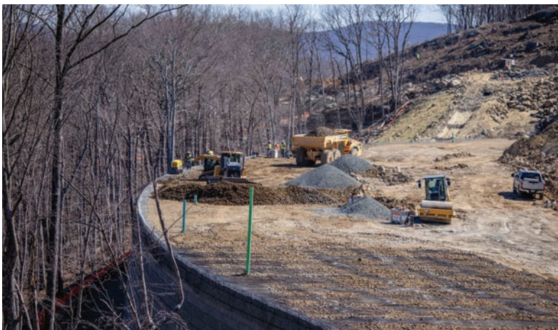
MSE wall under construction, showing reinforcement layers, wall facing, and backfill
